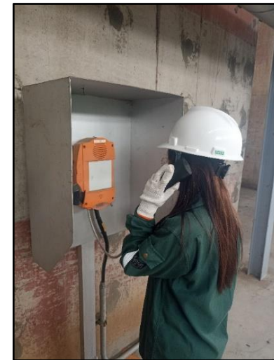
Checking and testing of inter-com system.
