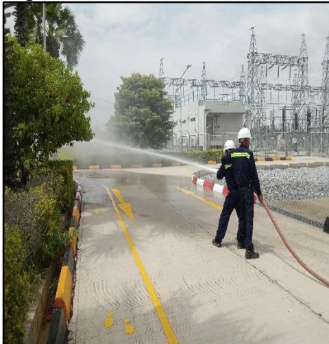
Fire hydrant and hose inspection and testing
