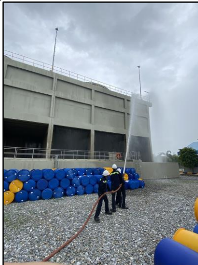
Fire hydrant and hose inspection and testing
