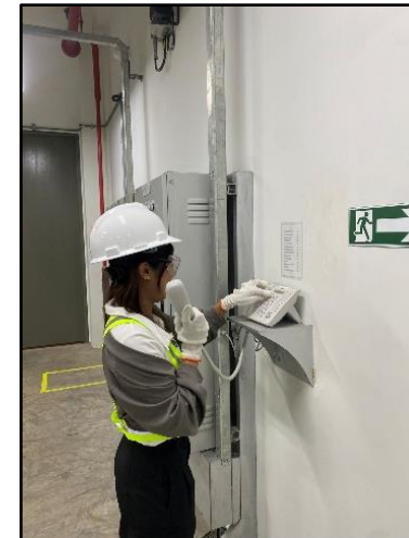
Checking and testing of inter-com system.
