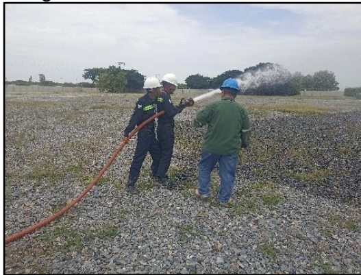
Fire hydrant and hose inspection and testing
