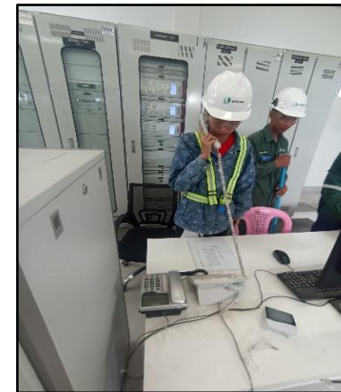
Checking and testing of inter-com system.
